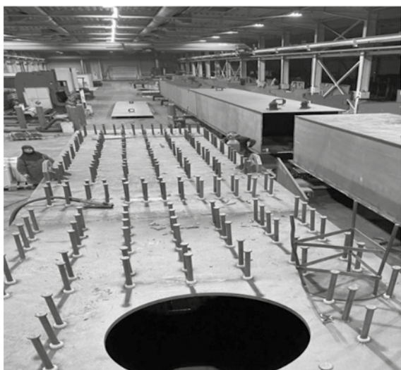
Figura 4. Segmente de pod rutier; grinzi cheson Figure 4. Road bridge segments, box section girder
