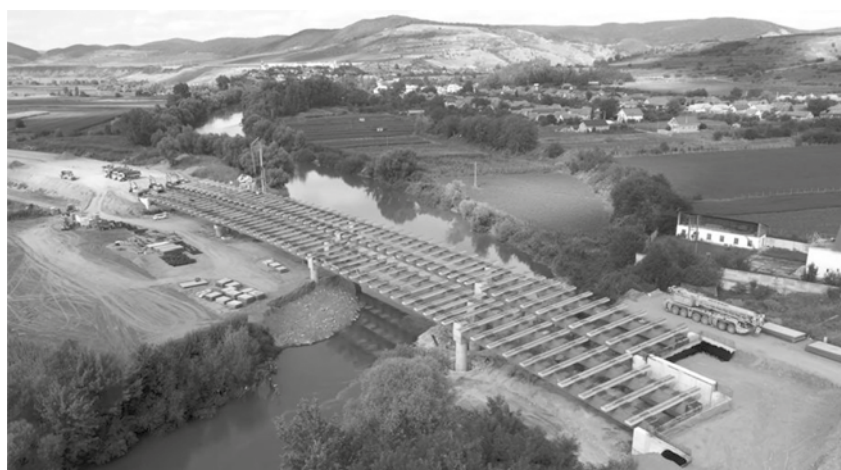
Figura 5. Pod peste Mureș, lungime L = 268 m – autostrada Sebeș – Turda (2020) Figure 5. Bridge over Mureș, length L = 268 m – highway Sebeș – Turda (2020)
